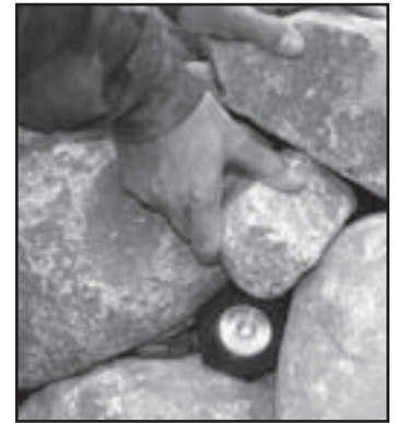
Fig. 20 Set your underwater lights in between your boulders so they are hidden from view.
