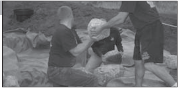
Fig. 18 Starting at the bottom, set the largest character boulders first then fill in with the smaller ones.
