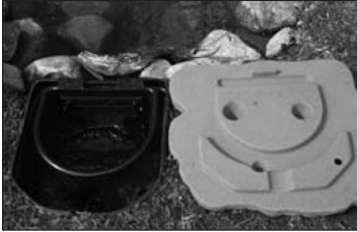
Fig. 34 Look at the underside of the stone to determine the proper interface with the shape of the skimmer basket.
