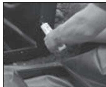
Fig. 15 Apply a bead of fish-safe silicone sealant around the skimmer opening, over the nut inserts.
