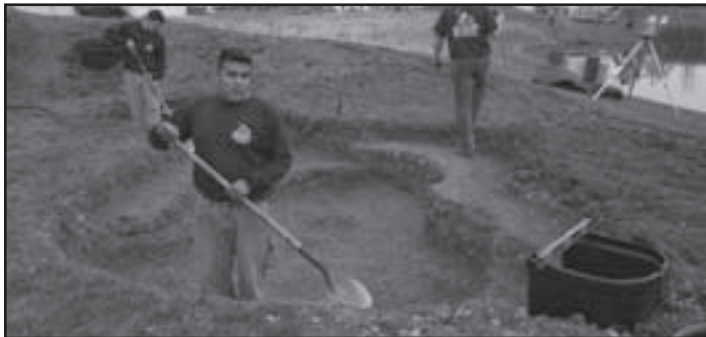
Fig. 6 Dig the pond to its max depth and finish excavation of the skimmer hole.
