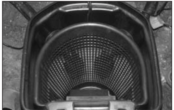
Fig. 31 Place the basket in the skimmer.
