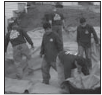
Fig. 9 Place the liner on top of the underlayment following the same installation procedures. Make sure liner is positioned in such a way that allows it to extend and completely cover the opening on the BIOFALLS® filter.
