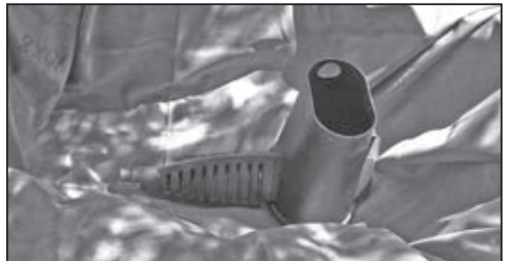
Fig. 7 Place the MicroSnorkel™ and MicroCentipede™ on top of the liner.
