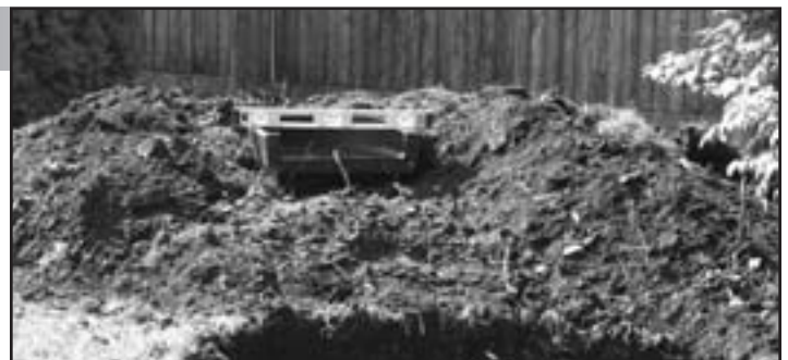
Fig. 5 Soil backfilled around the BIOFALLS® filter helps hide the filter and creates a planting berm.
