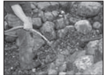
Fig. 22 Set larger boulders (6" – 18") around the perimeter of the basin.
