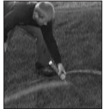
Fig. 1 Spray paint and outline the shape.
