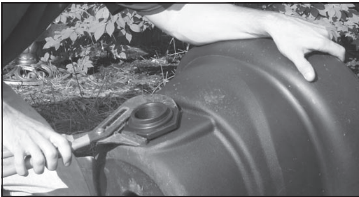
Fig. 1 Attach bulkhead fitting.
