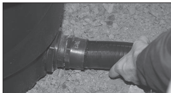
Fig. 4 Finished bulkhead assembly.
